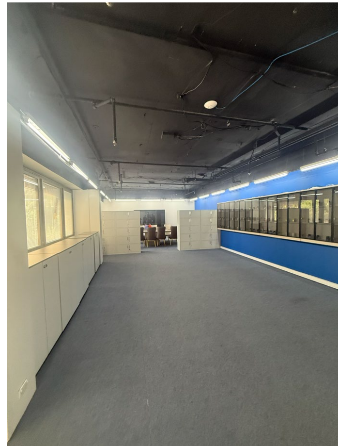
existing ground floor facing north
